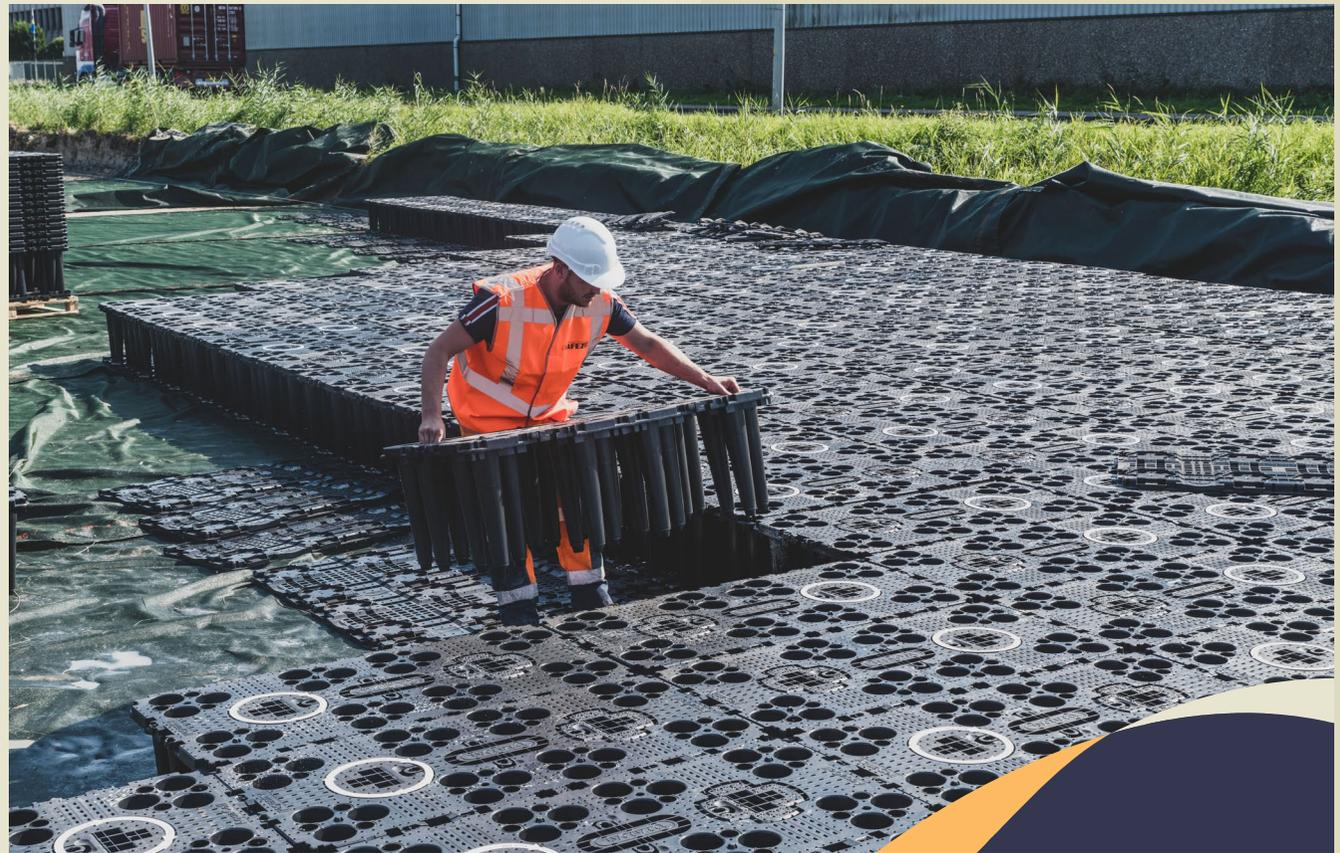
AquaCell infiltration tank made from 100% recycled material
